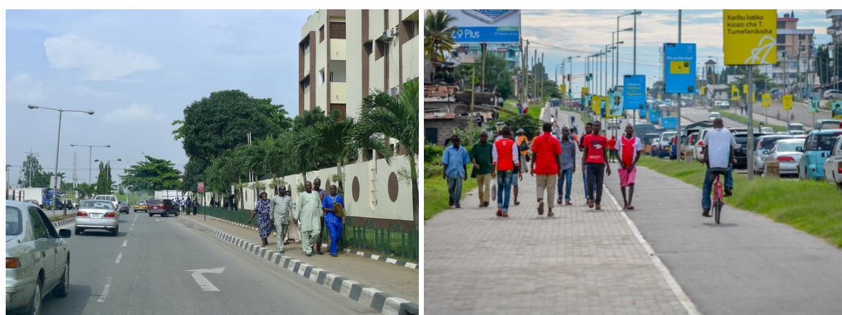
Figure 5: All streets should have safe, continuous space for pedestrian movement (left). Dedicated cycle tracks are an important component of a complete cycle network (right).
