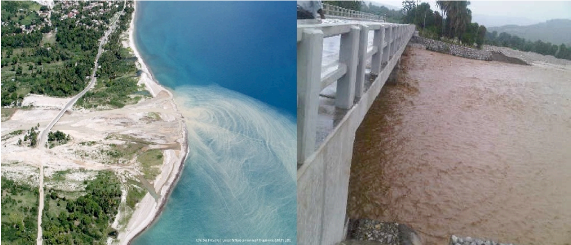
Figure 11. River discharge from Port-à-Piment (left). Flooding in the same area, in April 2012 (view from the bridge). Photos from UNEP.
