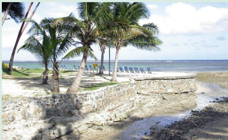
Figure 9.14 Coastal erosion and sea wall protection on a beach in Fiji
