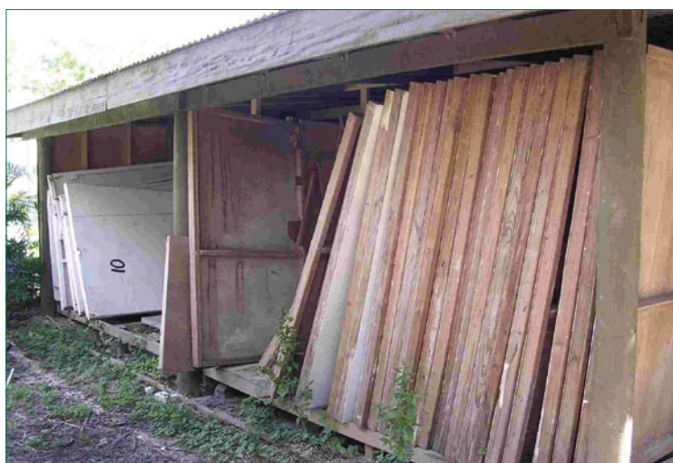
Figure 9.10 Windows shutters as a protection against hurricanes
