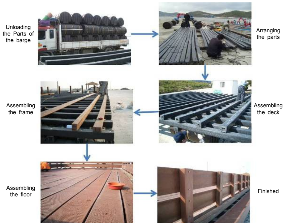
Figure 2. Process of building a floating receptacle for marine litter.
