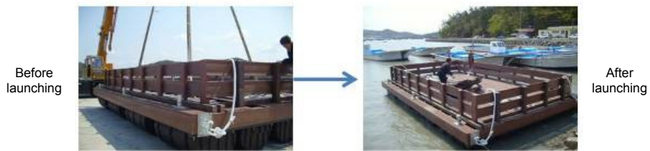
Figure 3. A floating receptacle before and after launching into port.
