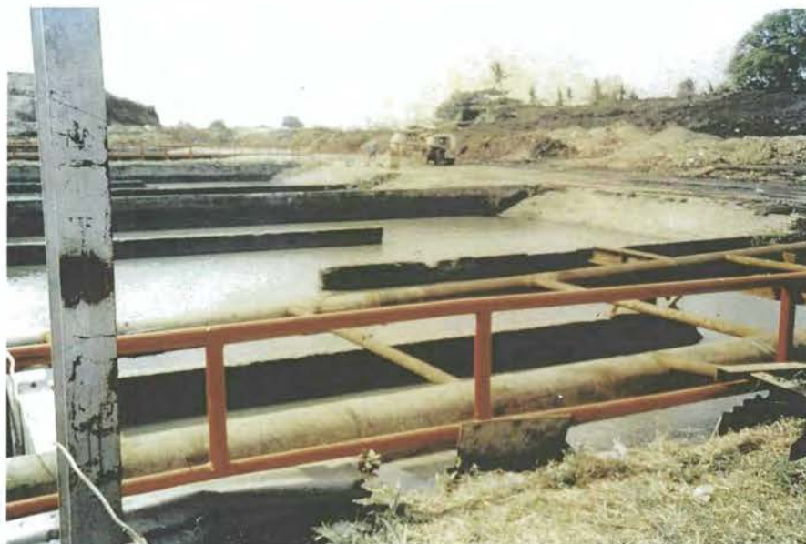
Ash settling pond
