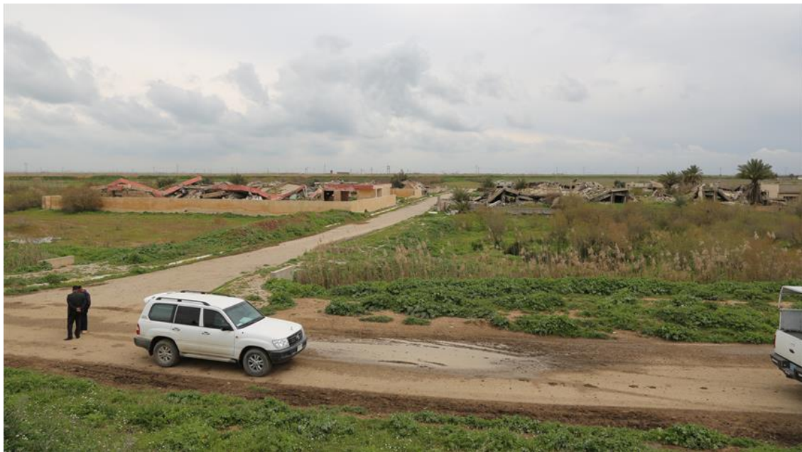
Photo 1: Typical damage to homes in villages in rural Kirkuk where an estimated 9,400 homes have been destroyed.
