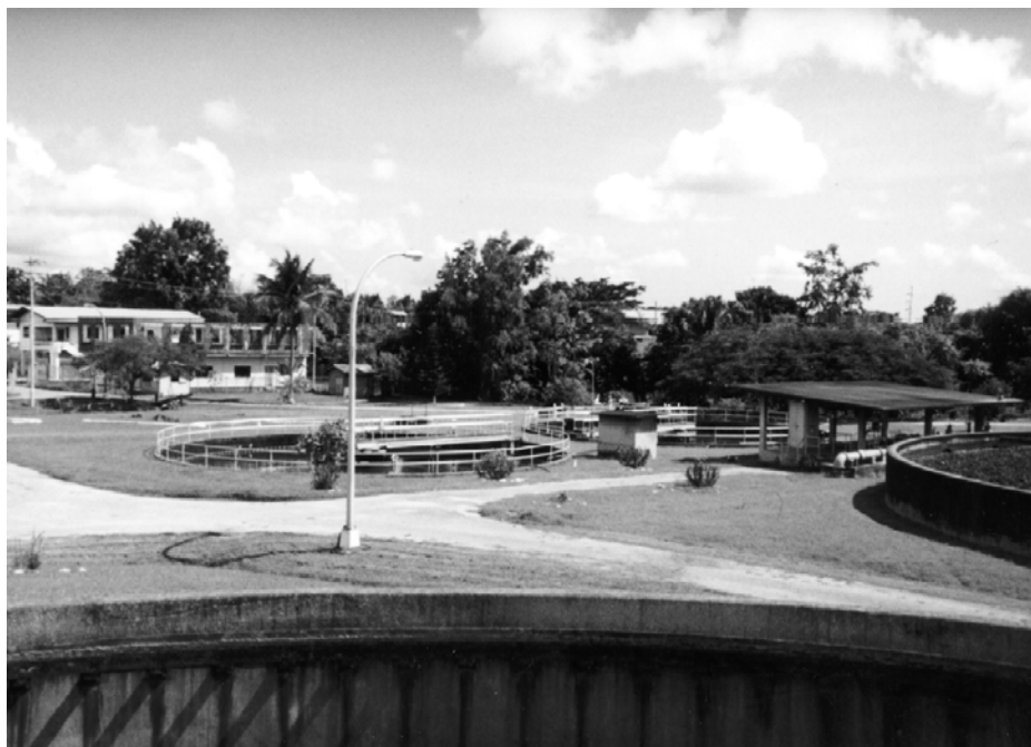
The San Fernando sewage treatment works.
