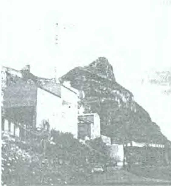
An Incinerator in Gibraltar (Credit: Warmer Bulletin)
