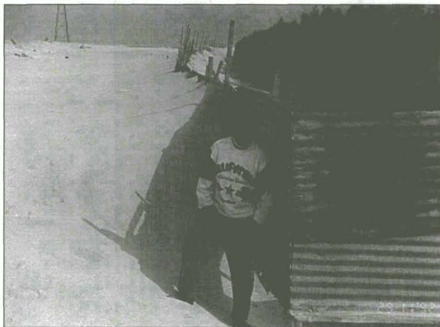
Figure 5: Sand fence (solid corrugated plate), closely spaced from the Tamarix aphyllae trees (western side, Al Wafra farms).
