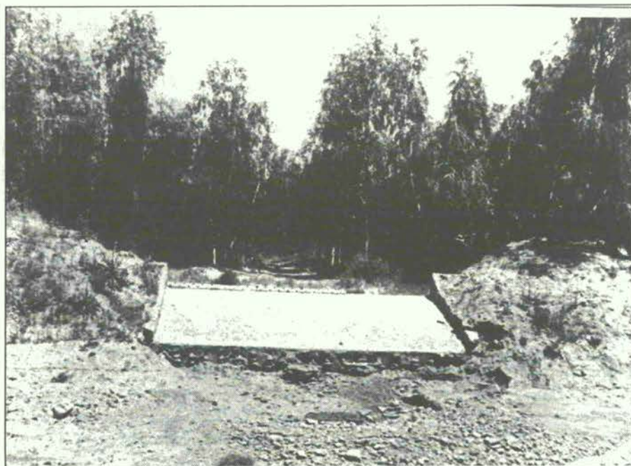
The eight year old trees in the Sedimentation Basins
