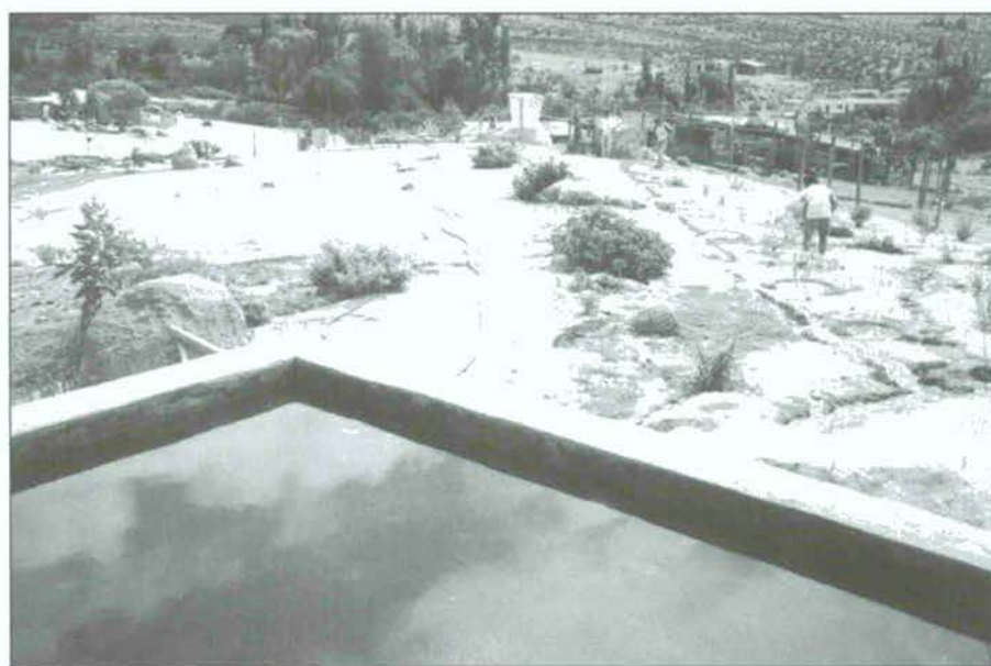
Photo 1. Cement tank for water storage.
