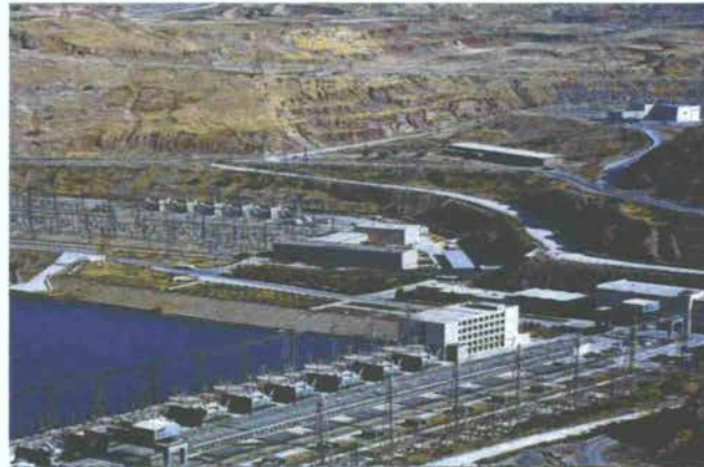
Fig. 22. Nurekskaya HPS, dam height 300 m
