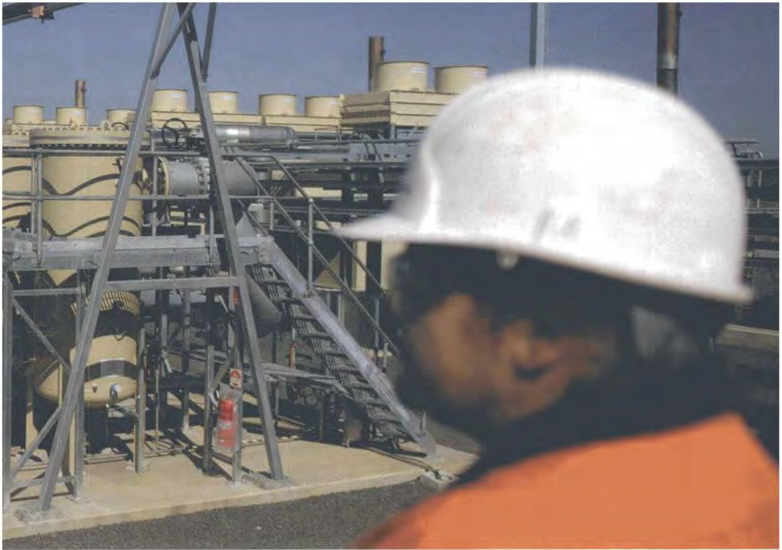
North mine. The plant generates electricity from methane-rich gas that is released during underground mining operations. The plant is owned and operated by Energy
