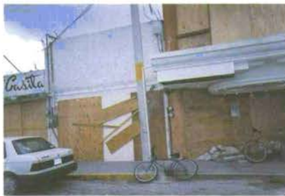
Getting ready for hurricane Mitch on the island of Cozumel, Sergio González Bucio, Mexico
