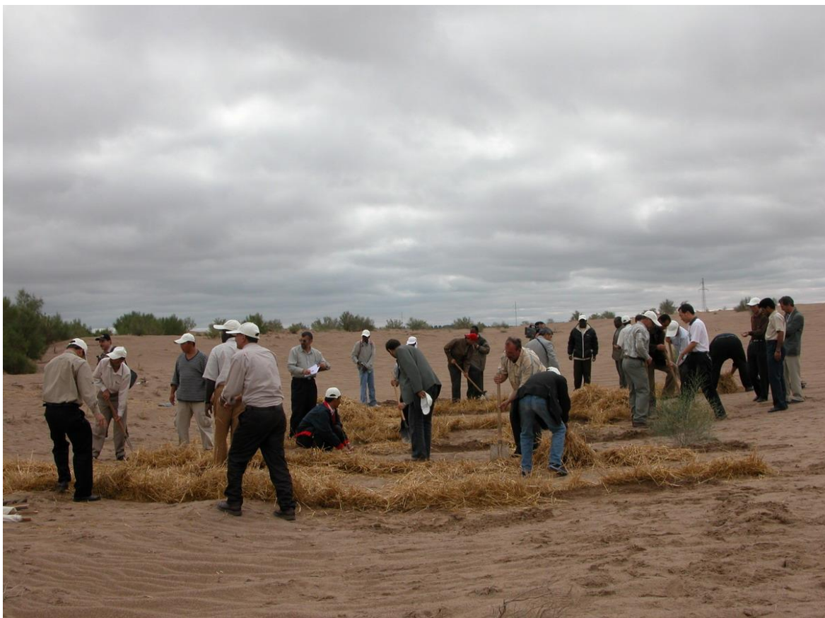
Figure 7 Trainees Participate in the Practice of Desert Control Grass Grid Laying
