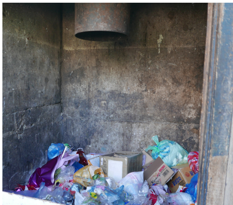
A waste chute in an older apartment building in Ulaanbaatar. Photos by Joni Seager.
