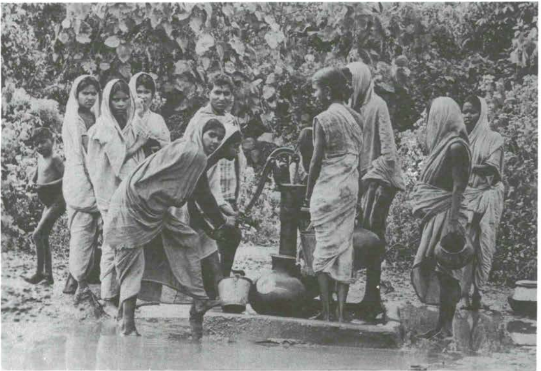
FIGURE 4-3 HAND PUMP WITH INADEQUATE DRAINAGE
