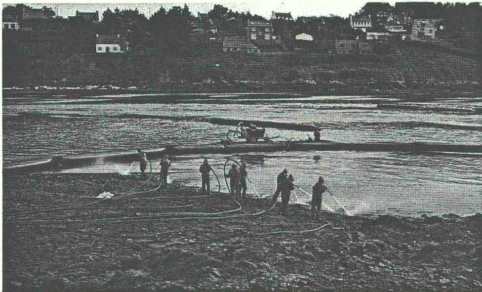
1. Curtain boom used to contain oil released by shoreline clean-up.
