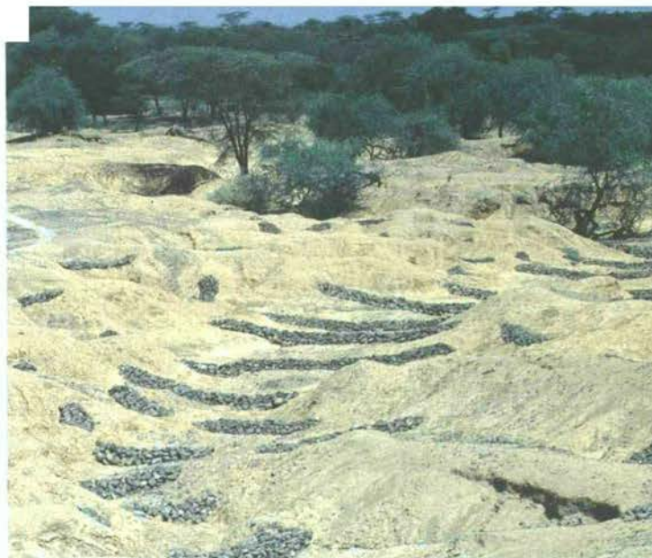
Check dams made up of stones serve to catch eroding silt behind them when water flows, thus filling up the gullies. (UNEP/Daniel Stiles)
