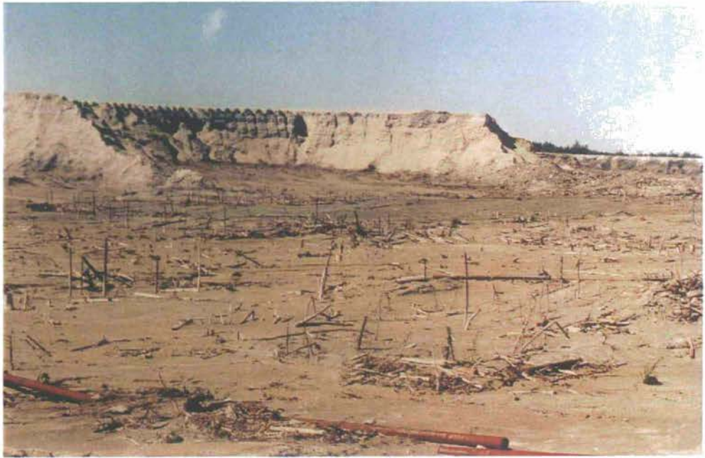
Picture 3 : Tailing dam failure showing destruction of a wooded area by earth flow.
