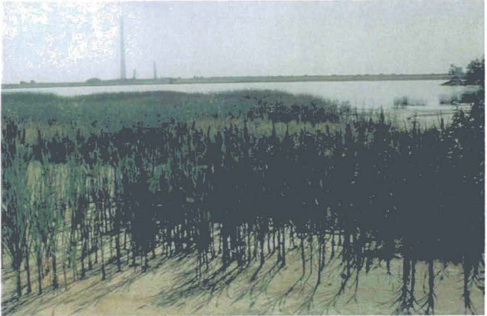
Picture 9 : Rehabilitation tailings using wetland technique which raises pH, causes heavy metals to precipitate to the bottom and provides habitat.
