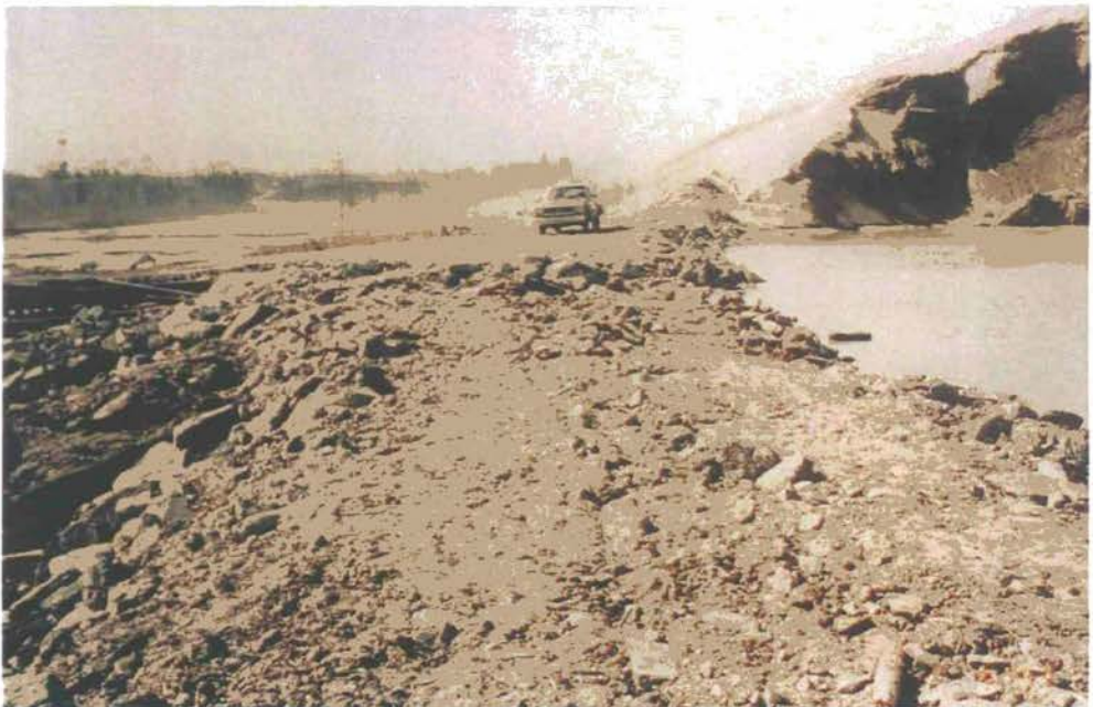
Picture 2 : Close-up of the emergency berm in photograph 1.
