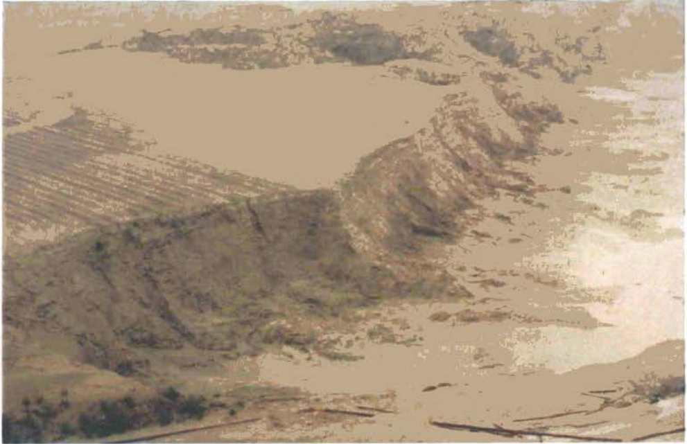
Picture 1 : Major tailings dam failure. In the foreground is an emergency berm used to stop the earth flow.
