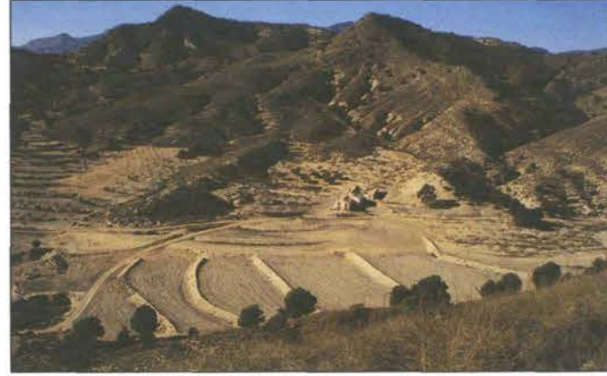
Figure 4.23 Area of marl and limestone affected by drought and overgrazing during the last decade
