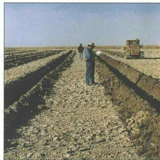
Figure 4.56 Constructing summer flood diversion channels
