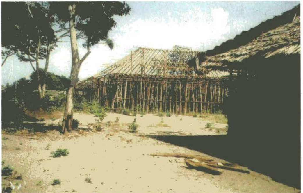
The framework of a traditional house made of mangrove poles
