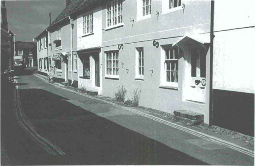
Figure 64 Cottagers in Bosham have adapted their doorways by raising the threshold steps to keep out the recurring sea floods
