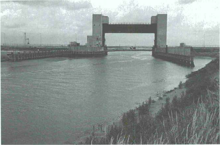
Figure 62 On the Darent River, a tributary of the lower Thames, storm surge flooding can be excluded by lowering a gate to close the river channel
