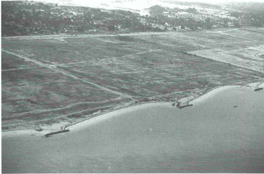
Figure 57 The southern coast of Singapore Island was advanced by extensive land reclamation in the 1970s. Segments of sea wall were built in the hope that the intervening beach sectors would become adjusted to prevailing wave patterns, and attain stability. However, erosion has continued, and the wall segments have been lengthened
