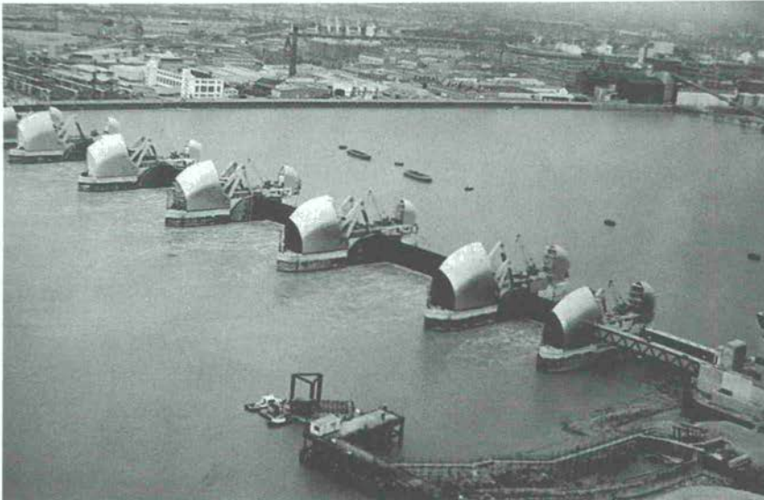
Figure 61 The Thames Barrier, completed in 1983, has rotating gates that can be raised to prevent storm surges raising the water level and flooding low-lying parts of London. Photograph reproduced by permission of the National Rivers Authority, Thames Region
