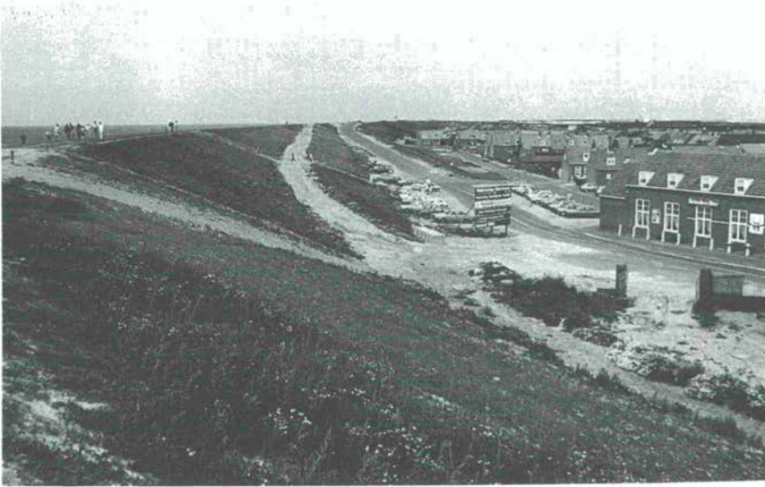
Figure 67 The sea wall at Westkapelle after its enlargement in 1987
