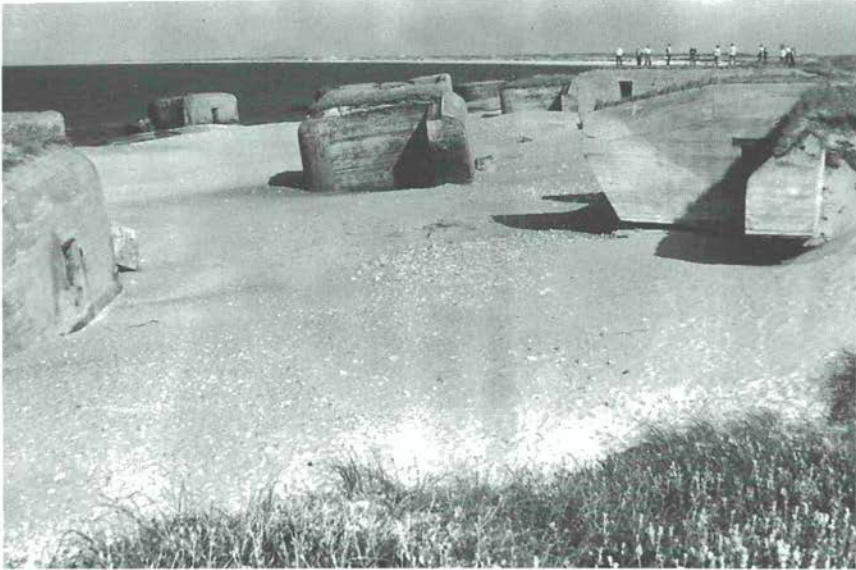
Figure 26 Beach erosion is extensive around the world's coastline. Here, on the southern coast of Jutland, Denmark, erosion has cut the beach back sufficiently to undermine defensive blockhouses built during the German occupation in the 1940s
