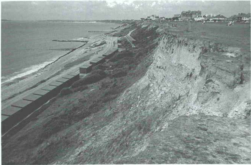
Figure 60 Cliff recession on the shores of Christchurch Bay, southern England, has been halted by the construction of a sea wall and esplanade, and the renourishment of the shingle beach. Cliff-crest recession continues, but the cliff is developing into a more gradually sloping bluff, which is expected to stabilise. As sea level rises it will be necessary to raise the level of the sea defences in order to prevent renewed erosion and further cliff retreat
