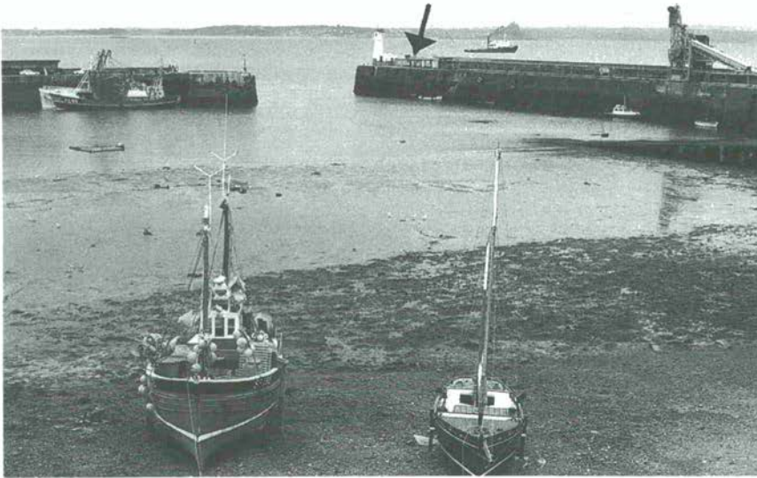
Figure 3 The tide gauge at Newlyn Harbour, in Cornwall (south-west England) is located in a building (arrowed) on the southern quay, near the lighthouse. It was used to establish mean sea level for the period 1915–1921 as Ordnance Datum for British topographical surveys, but by the 1960s mean sea level had risen 0.12 m here, an annual average rise of 2.4 mm per year
