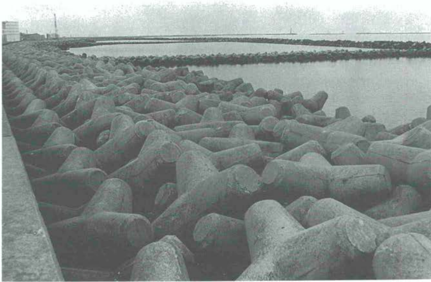
Figure 71 Land subsidence at Niigata, Japan, indicated in Fig. 70, resulted in the disappearance of the beach and the subsequent armouring of the coastline with large concrete tetrapods and breakwaters
