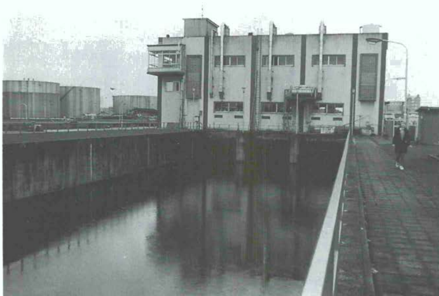
Figure 72 Pumping stations are necessary to keep low-lying parts of urban Niigata (Fig. 70) free from marine flooding and to remove floodwaters from the Shinano River
