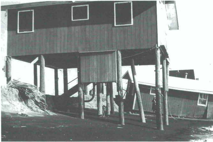
Figure 80 Beach erosion on Rhode Island, United States, has damaged and destroyed holiday shacks built on a barrier island
