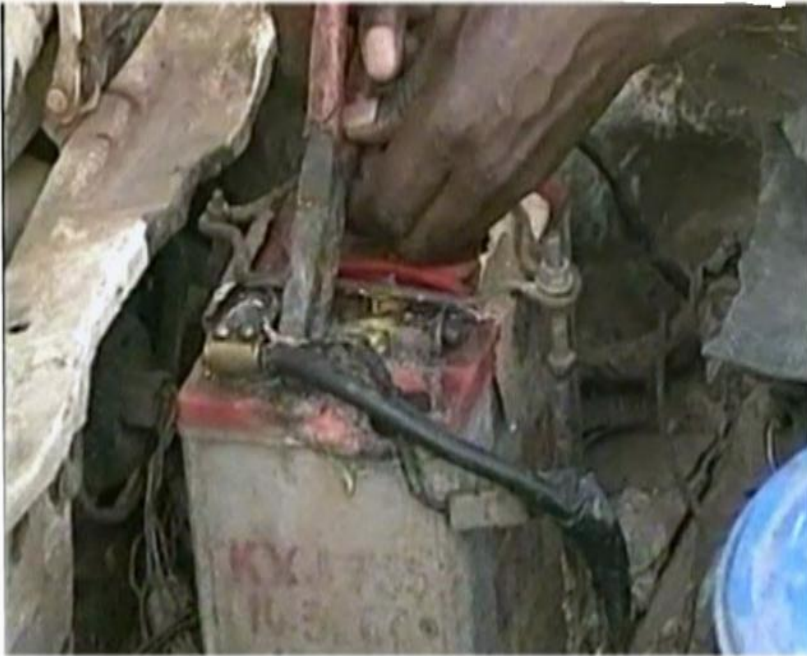
Dismantling of ULAB in open
