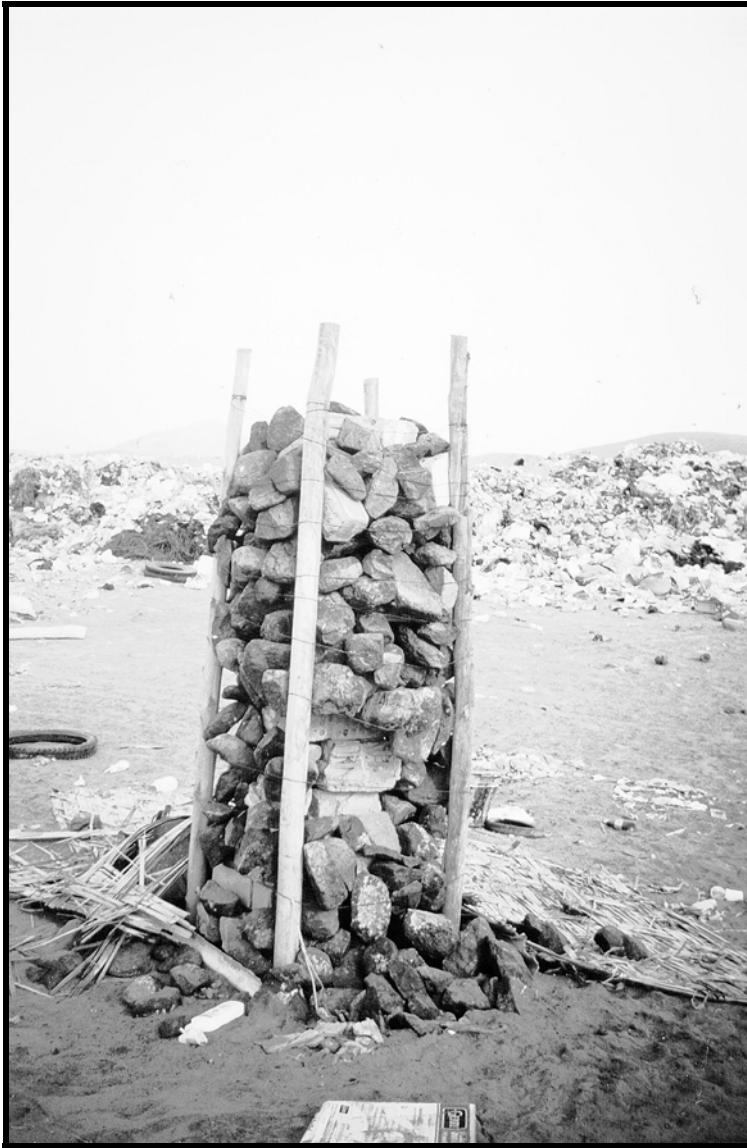
Figure XIV-22. Gas removal unit made with locally available materials
