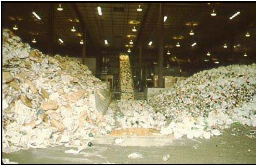
Figure VI-23. Example of a tipping floor and stored materials at a source-separated processing facility
