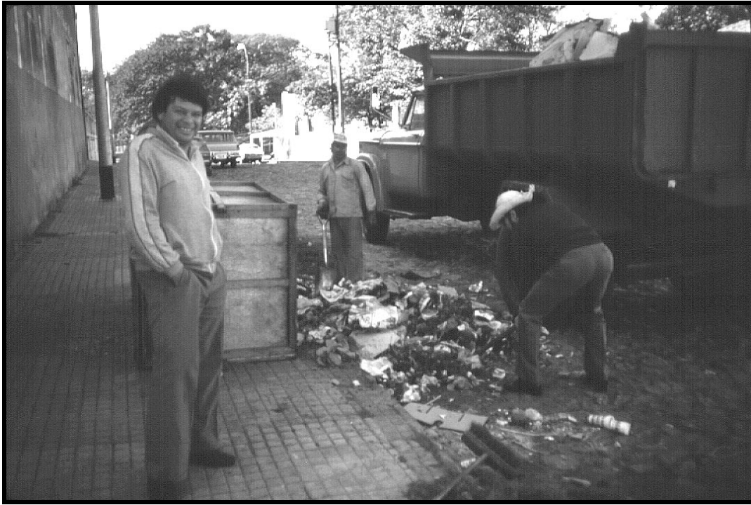
Figure IV-10. Emptying of wastes from handcart for reloading into larger collection vehicle
