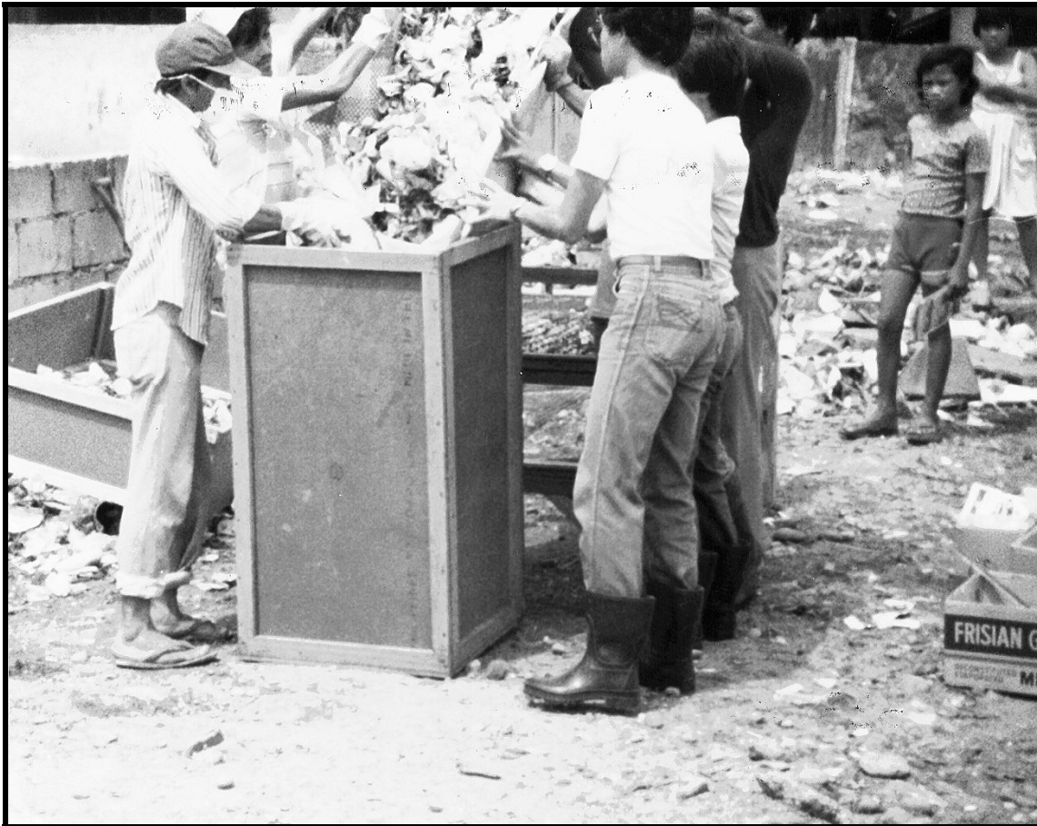
Figure III-11. Determination of bulk density
