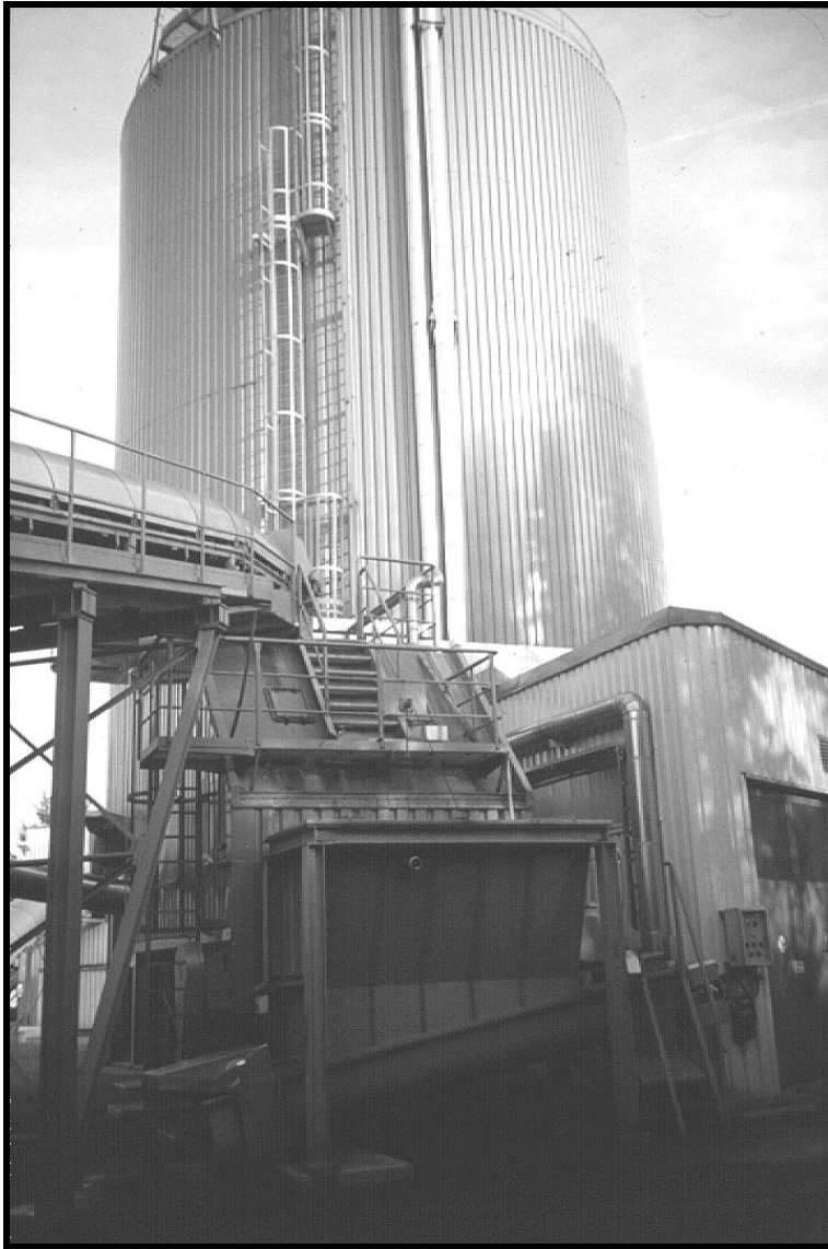
Figure XI-9. Example of high-solids anaerobic digester
