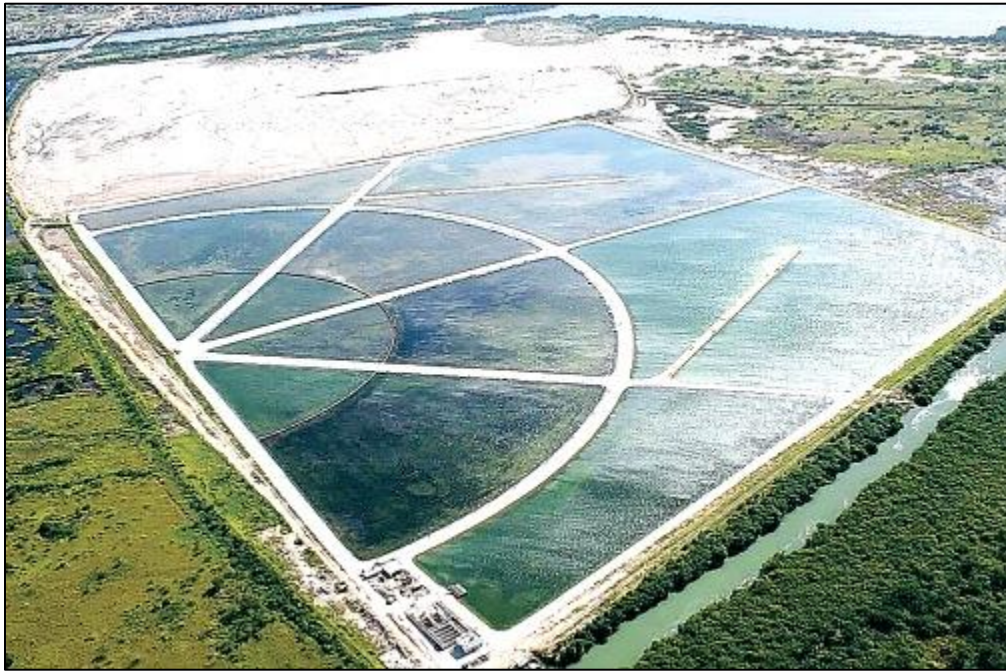
Figure 19: Soapberry Sewage Treatment Plant
