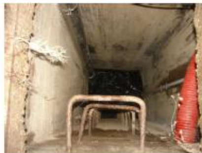
Wastewater Treatment & discharge
