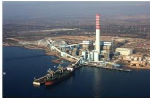
Coal-burning power plant
