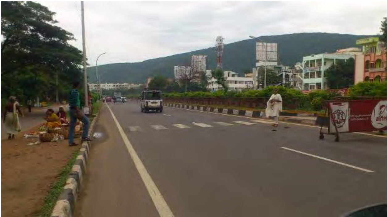
Figure 25 Inadequate street infrastructure along the NH-5
