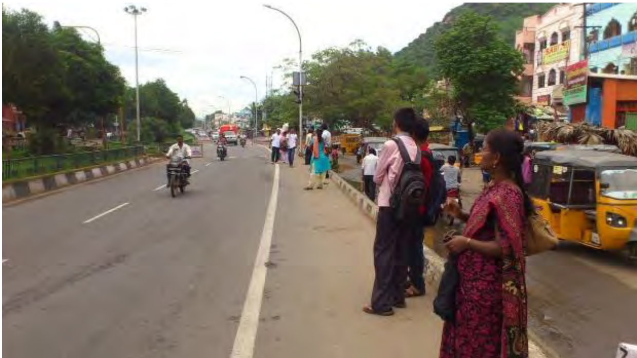
Figure 19 Inadequate bus stop facilities
