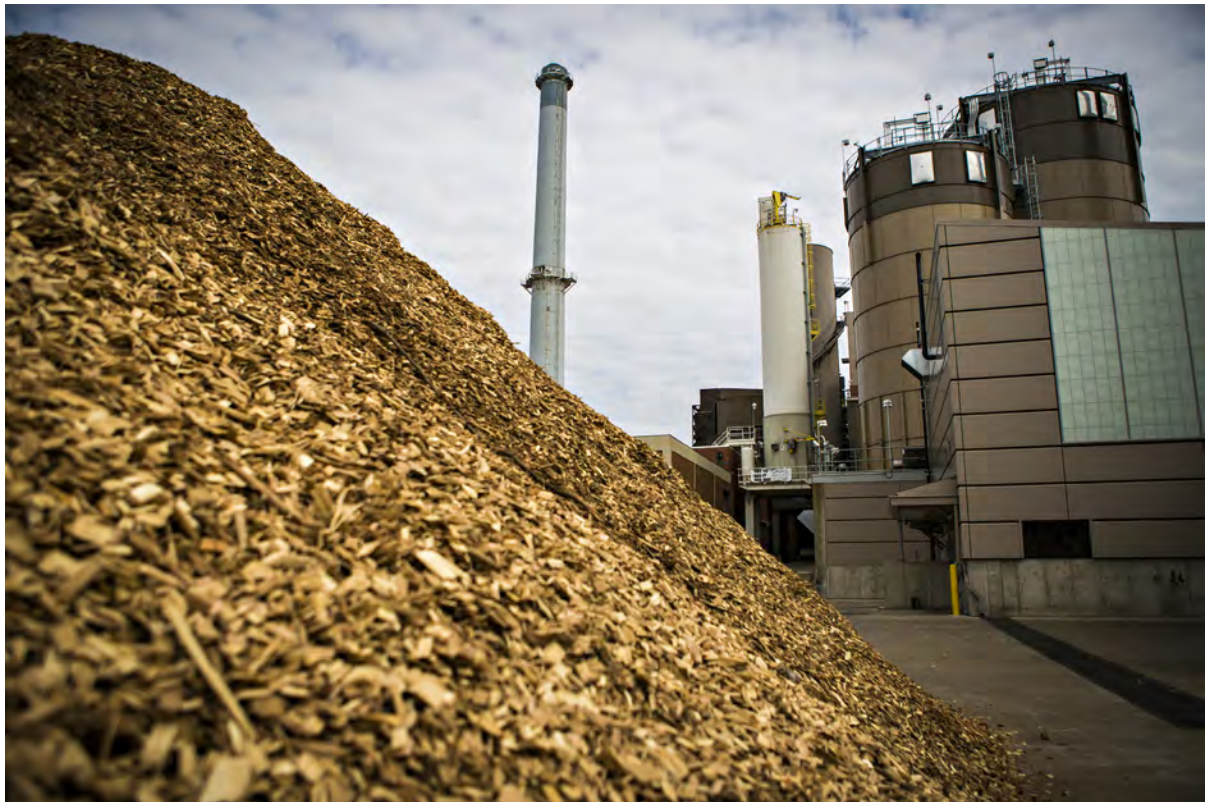
Photo of biomass boiler using grass and wood chips. Photo courtesy of Kyle Spradley, Curators of the University of Missouri, 2014. Info on the rights reserved: http://creativecommons.org/licenses/by-nc/4.0/
