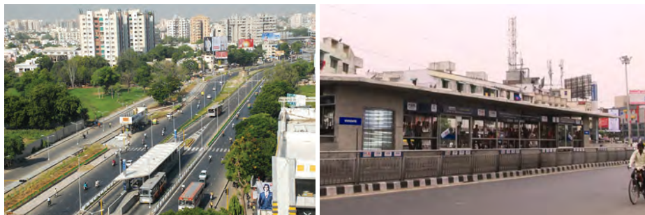
Figure 1: BRTS known as ‘Janmarg’ in Ahmedabad city
