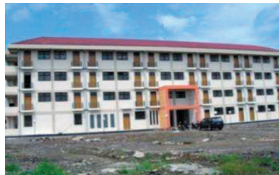
FIGURE 5.4 Bambe slum upgrade building in Indonesia (Government of Indonesia, 2012)
