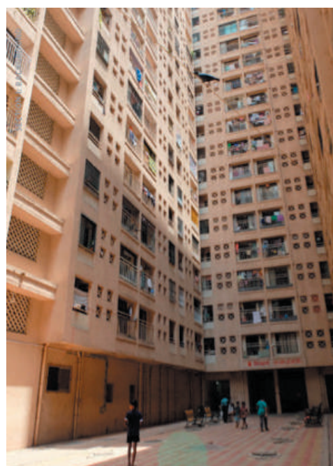
FIGURE 5.3 Multi-storey slum housing rehabilitation in Mumbai, India
