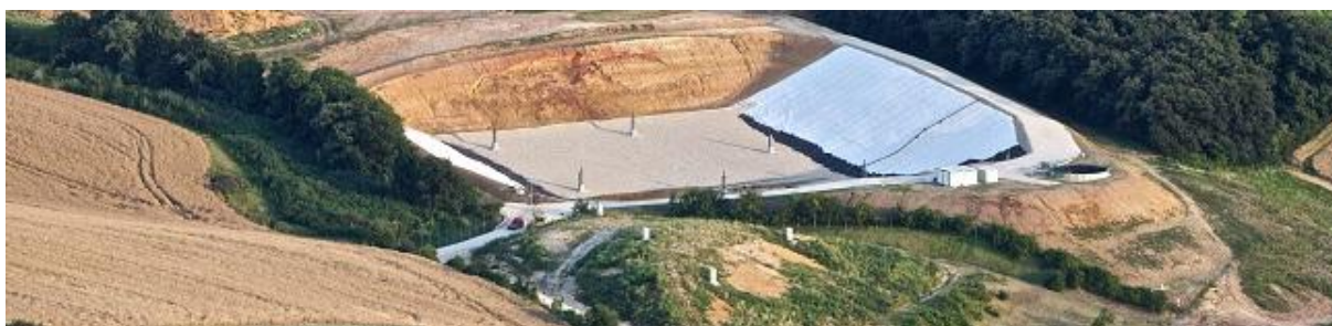
Picture 6: Landfill foundation
