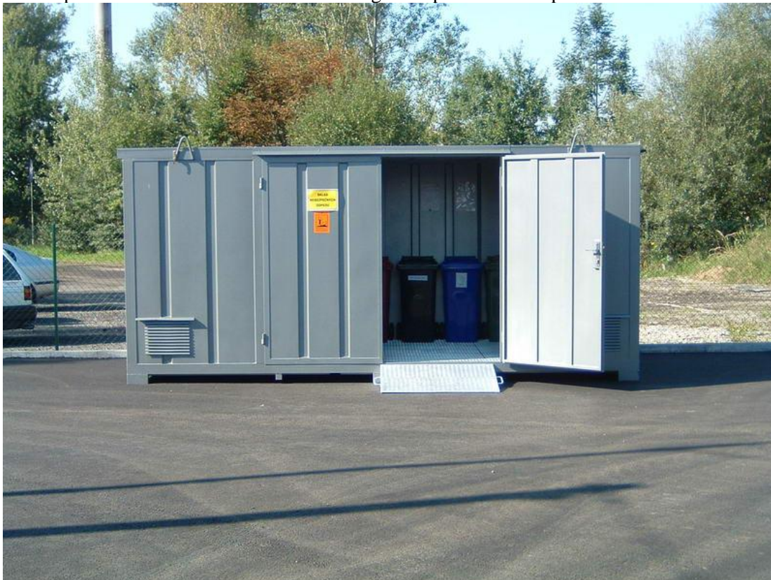
Picture 4: Mobile storehouse of hazardous wastes
