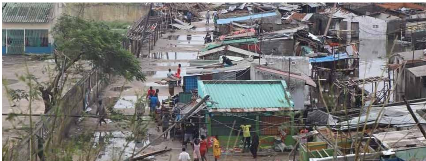
Destruction from Cyclone Idai. March 2019. Beira, Mozambique. (Photo credit: Beira Municipality.)
