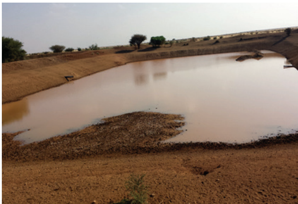
Water harvesting (hafir) for livestock in the Butana area © International Fund For Agricultural Development (IFAD)
