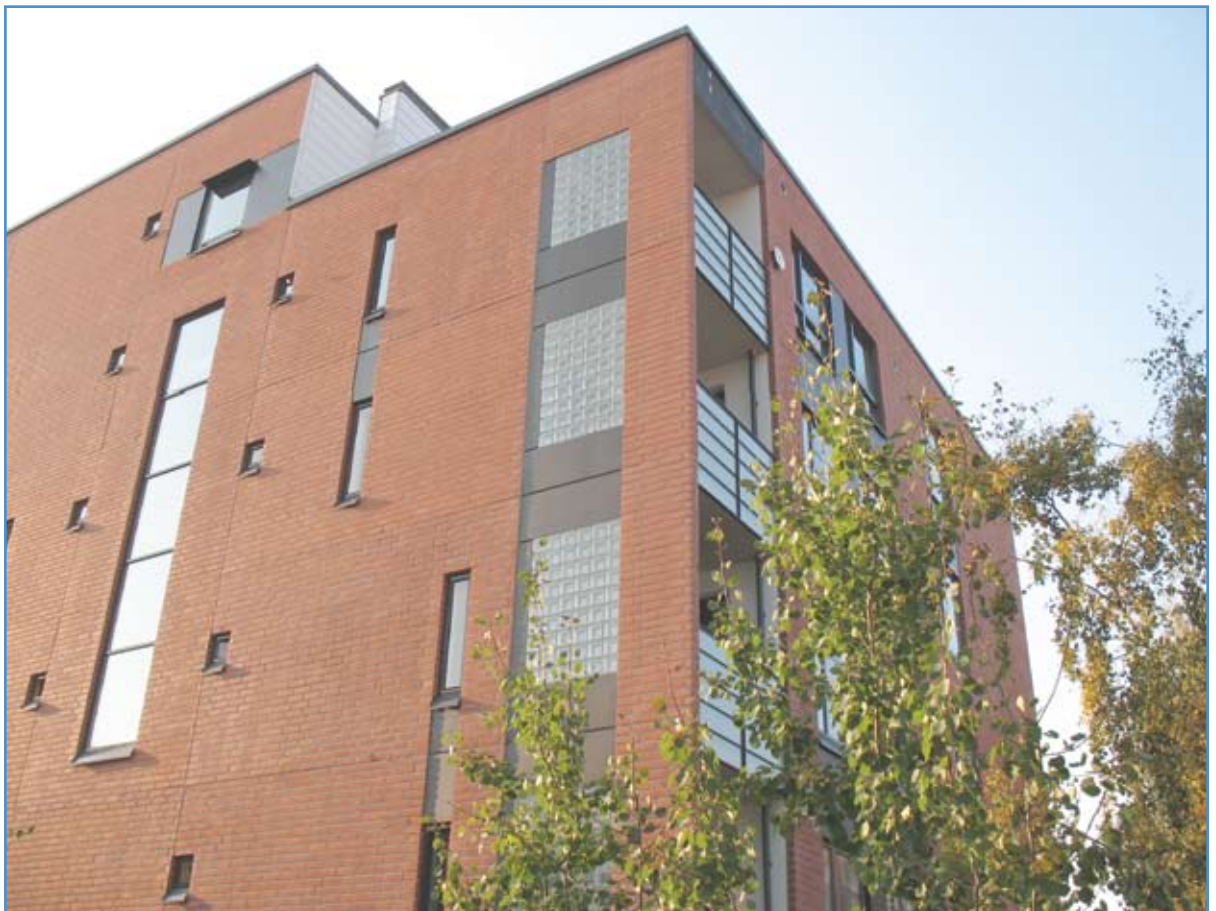
Figure 8. A passive apartment building in Finland. Photo: Mikko Saari, VTT
