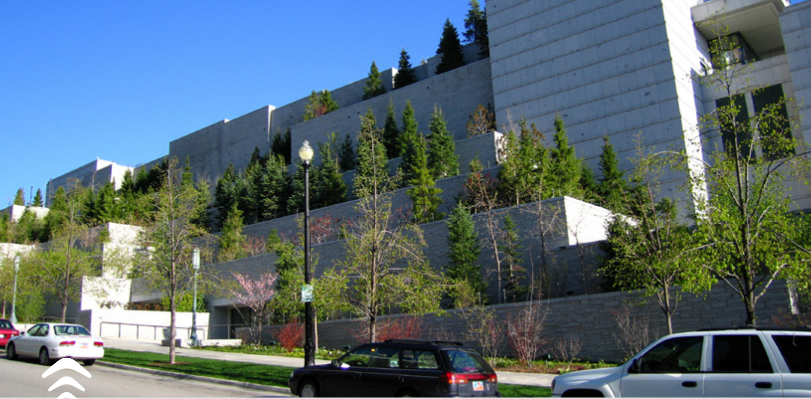
Figure 5.2. Green roofs can be used not only to enhance targeted ecosystem services, such as storm-water retention and food production, but also to improve biodiversity in general. For example, using local seed mixes and substrates can mitigate habitat loss and fragmentation and also enhance habitat provision and connectivity, when placement and height of the green roofs complement and support existing ecological communities in the surrounding landscape. Wildflower meadows (Salt Lake City, USA), nesting sites for birds (Basel, Switzerland), and invertebrate-rich “brownfields” — well-drained, nutrient-poor environments on previously developed lots (London)—are just a few examples of ecological environments created by green roofs. Large-scale rooftop agriculture initiatives already exist in many cities around the world, among them New York, Chicago, Singapore, and Montreal (see p. 38). Shown here is the roof of The Church of Jesus Christ of Latter-day Saints Conference Center in Salt Lake City, Utah.
