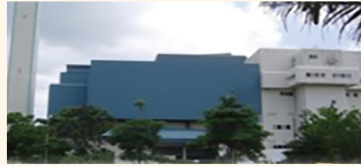
Stoker Incinerator Plant [No. 1] Capacity: 250 tonnes/day, stoker type Initial cost: THB 780 million Annual operation: 7,000 hours
