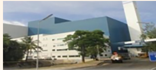
Stoker Incinerator Plant [No. 2] Capacity: 350 tonnes/day x2, stoker type Initial cost: THB 940 million Annual operation: 7,000 to 8,000 hours
