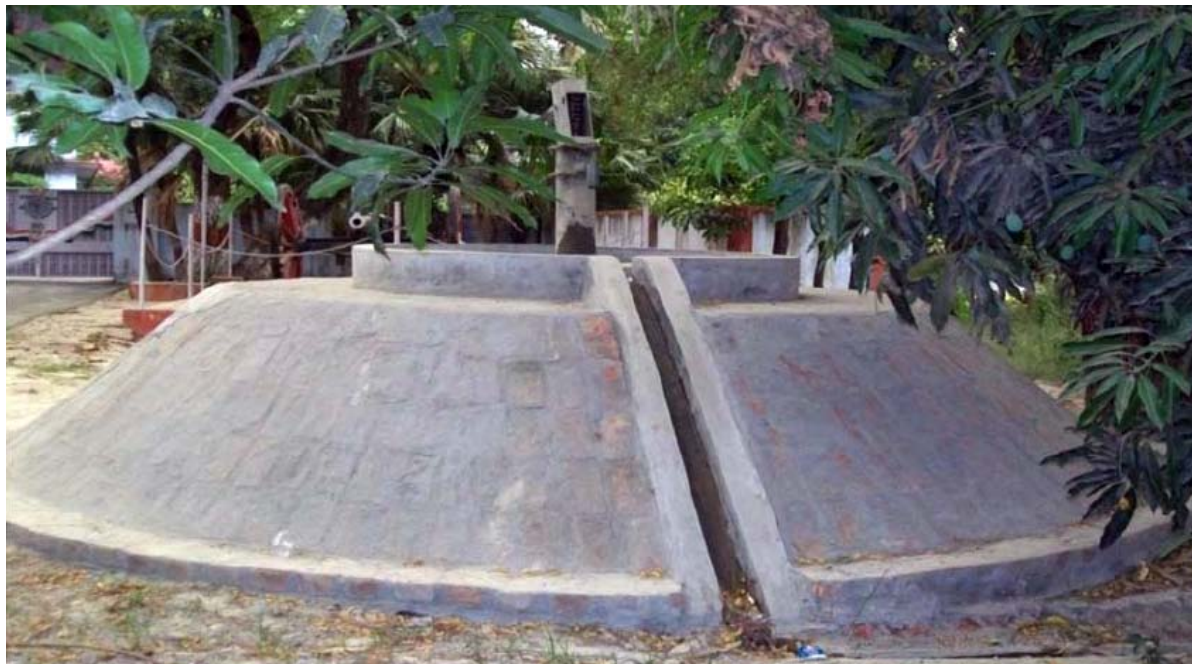
Figure 7: Flood-proofed handpump in Bahraich, Uttar Pradesh, India. The apron is 1-m high, 2.9-m in diameter. The slope of the base is 45-degrees, gradual enough to prevent damage to the base during flash flooding.
