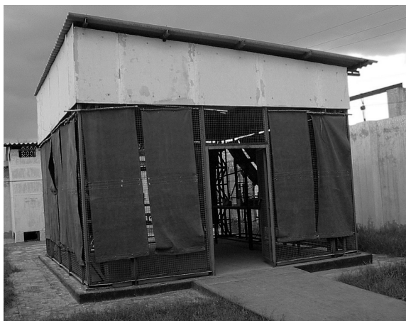
Example # 1: an undersized open air gassing room.
