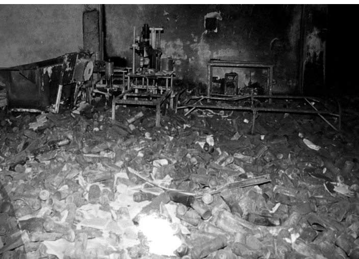
A solvent fire precipitated this havoc, which killed several workers, but the principal damage was done by exploding aerosol cans.
