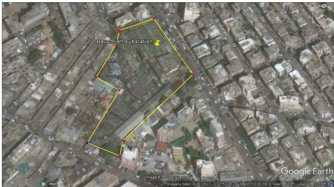
Figure C-5: Aerial view of Bauchrieh site
