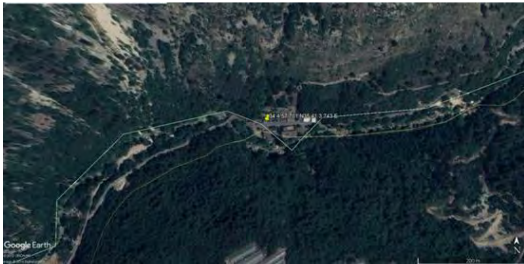
Figure C-13: Nahr Ibrahim hydro power plant
