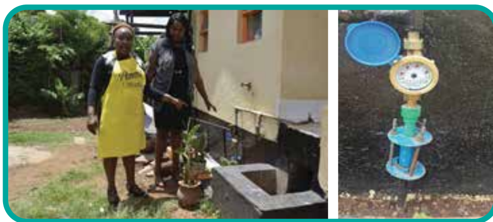
Pamat foods sub meter for the processing unit.
