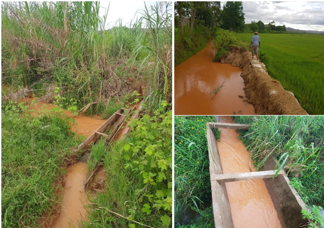
Figure 5. Irrigation canal and water infrastructure in Manakambahiny.
