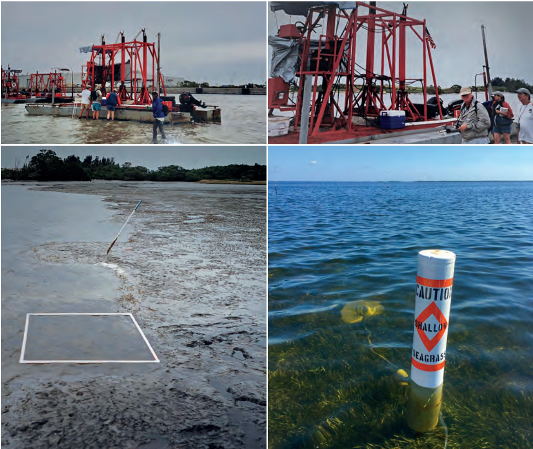
Plate 6. Seagrass salvage and restoration work at Tampa Bay (Florida): Top: 'Giga-unit sod' transplanting machine. Bottom (left): intertidal area from where 1x1 m seagrass sods have been removed with the 'giga-sod' machine (see frame for reference of scale). Bottom (right): demarcation buoys used to prohibit all entry, transit, anchoring or drifting within restricted areas to allow seagrass to recover from boating damage.
