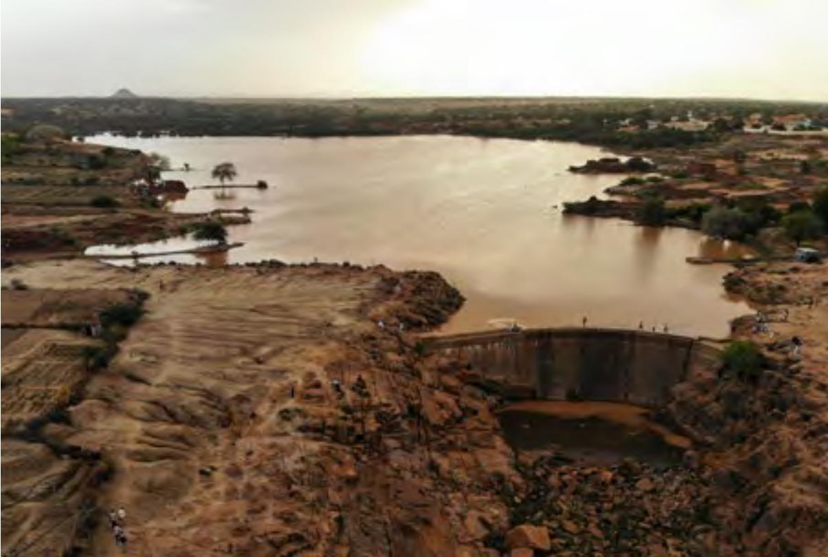
Water dam in Malit locality, North Darfur. Photo credit © UNEP
