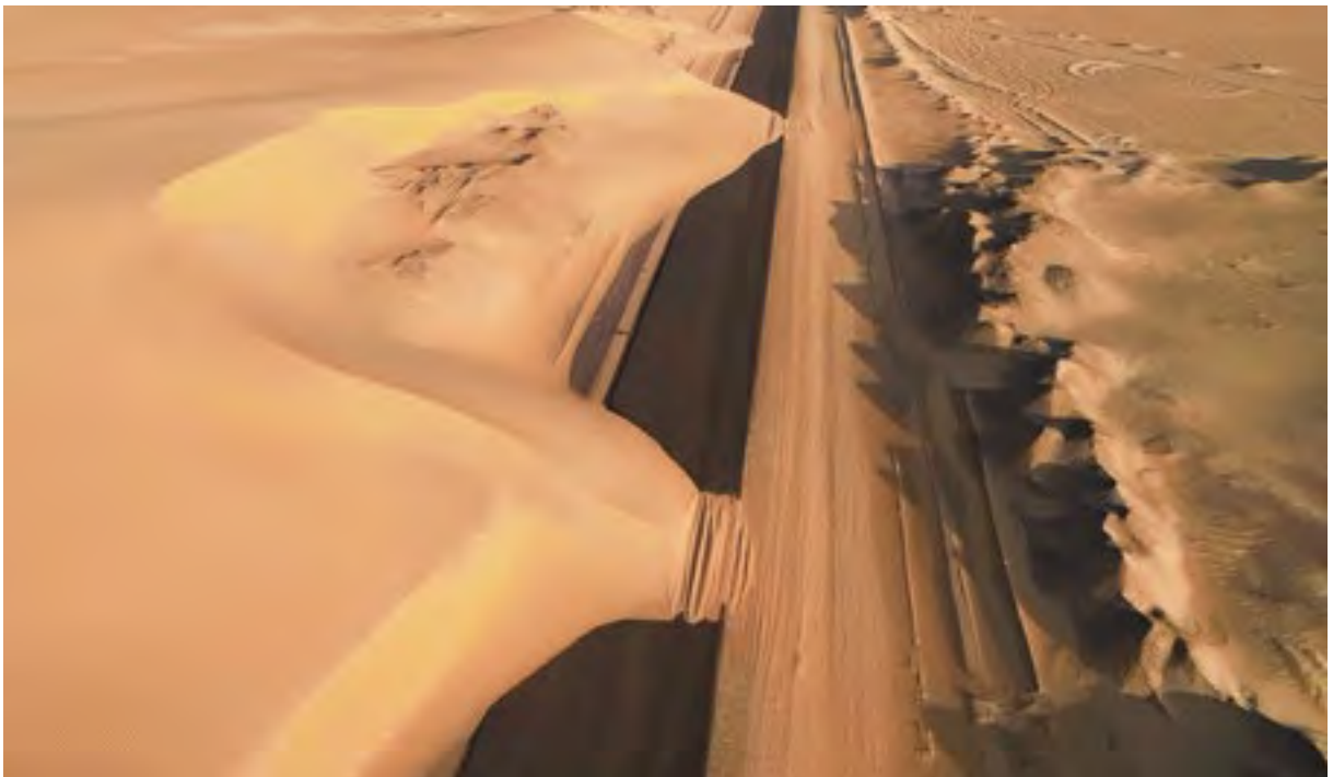
Sand movement obstructing major highway in Nawa, Northern Sudan. Photo credit ©UNEP
