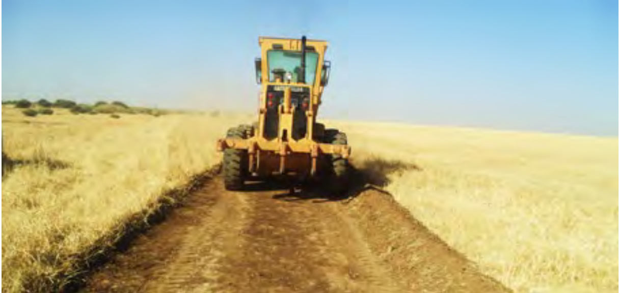
Opening of firelines is an effective method of decreasing the impact of fire on grazing lands. Photo credit © World Bank
