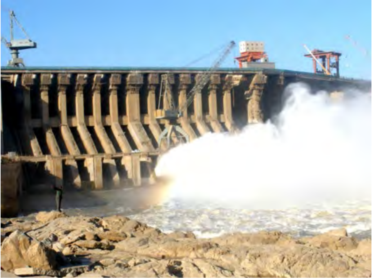
Merowe hydropower dam in Northern Sudan with a capacity of 1250 MW under hydropower generation. Photo credit © Osman Ali
