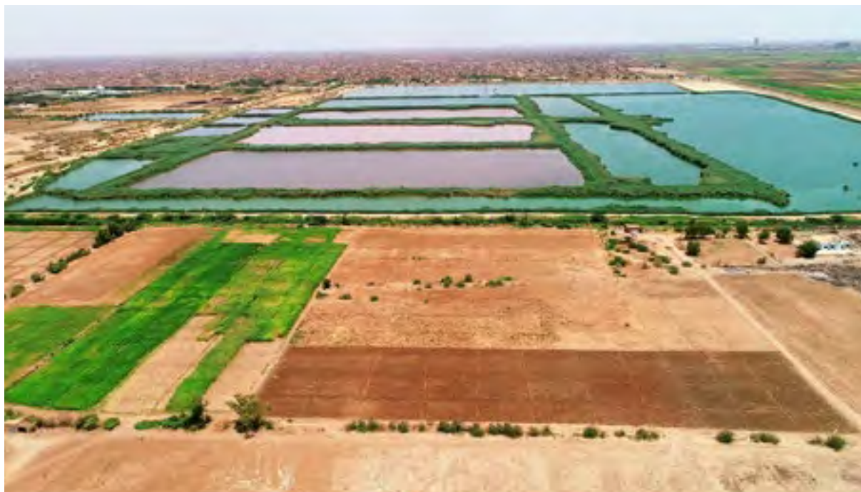
Domestic sewerage treatment plants in Khartoum State. Note the residential area in the background and the cropped area in the front. Photo credit © UNEP
