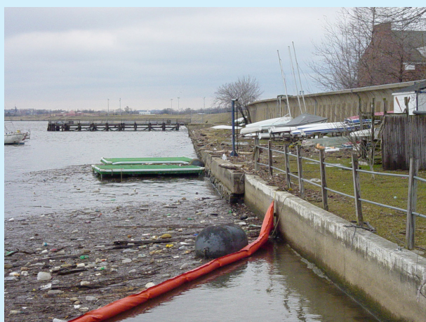
A boom system captures floating trash as it travels.
