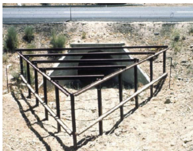
Figure 15. Upstream view of a steel debris deflector
