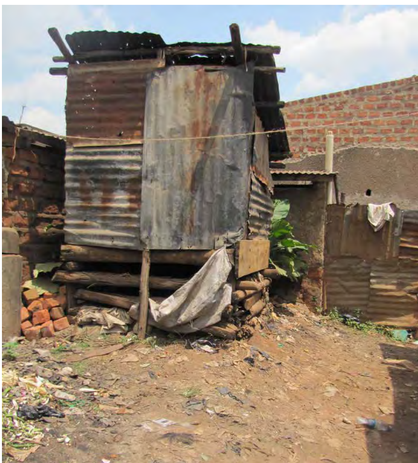
Open defecation is a result lack of basic sanitation facilities
