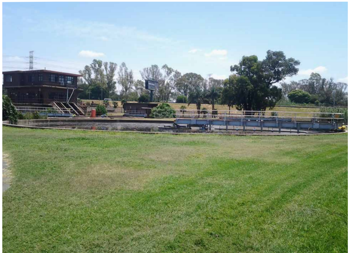
Reuse of wastewater to water lawns
