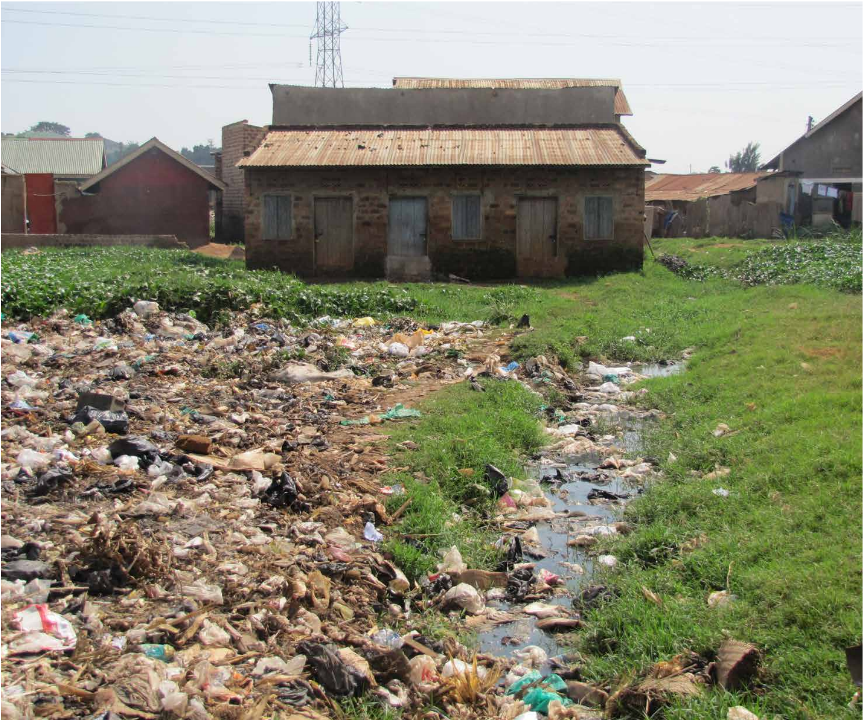
Sewage leaks and dumping of waste are common urban environmental hygiene problems in Africa
