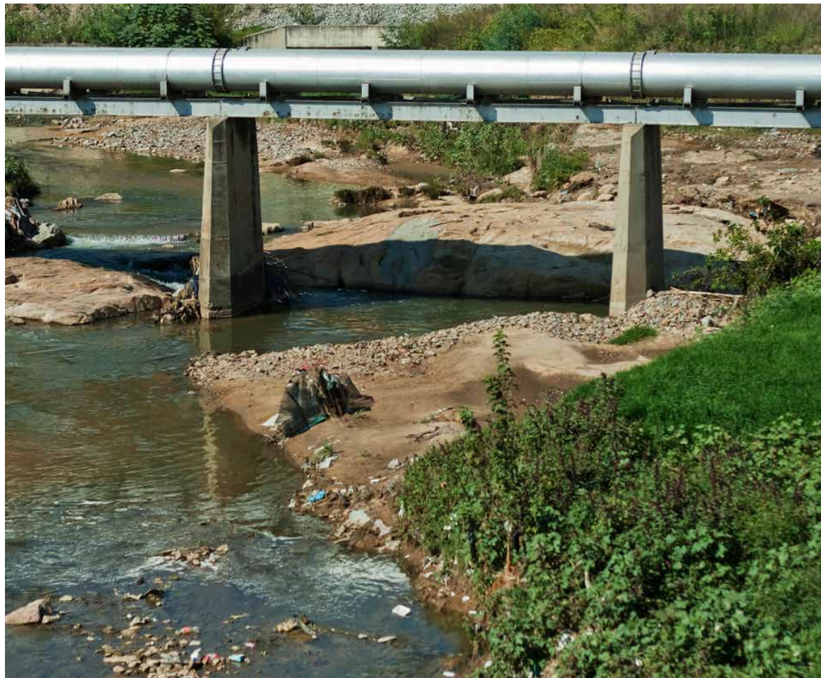
Off-site conveyance systems for excreta, faecal sludge and wastewater serve multiple households
