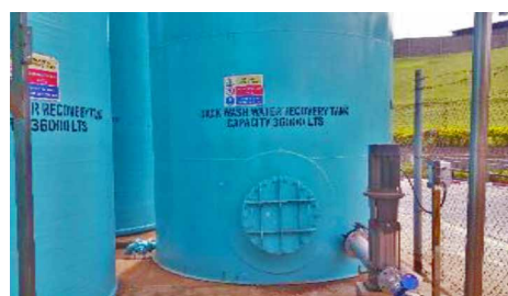
Backwash water which used to be sent to drain is now being recovered and reused
