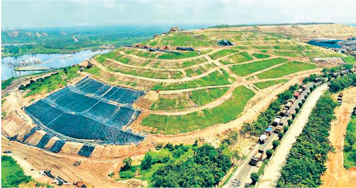
Figure 9.1 Capping of 135-acre Jawaharnagar dumpsite in Hyderabad (CSE, 2020)
