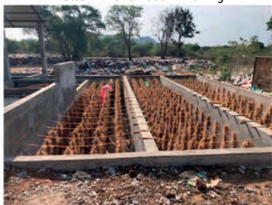
Leachate treatment system construction
