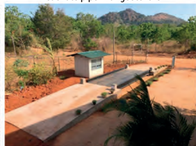
Weighing bridge construction
