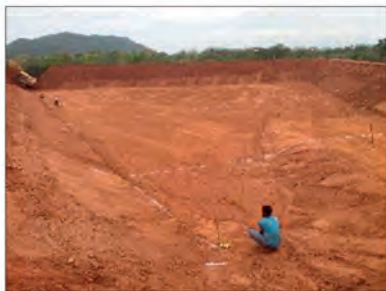
Bottom liner smooth finishing
