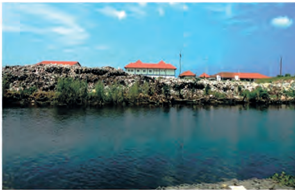
Dumpsite on a large canal
