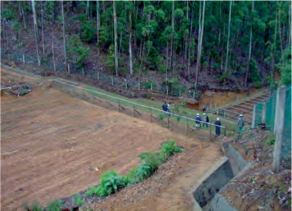
Moonplain semi-engineered landfill after rehabilitation (2004)
