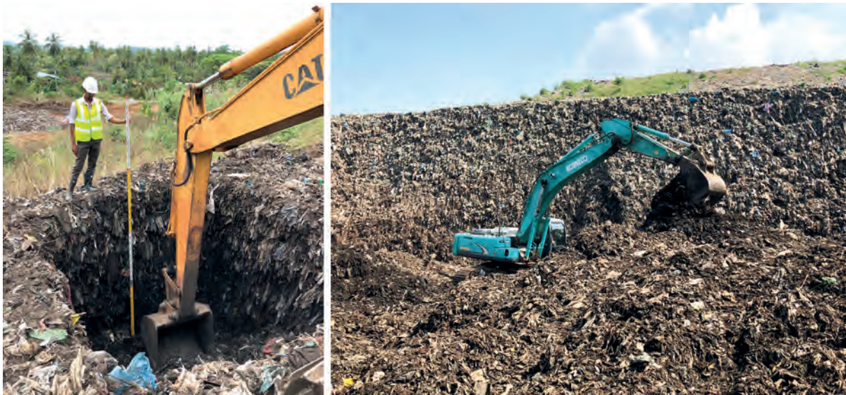
Figure 6.2 Assessing the potential of dumpsite mining by trial excavations
