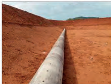
Leachate pipe installation
