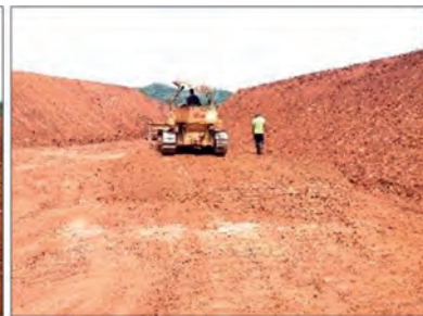
Bottom liner compaction
