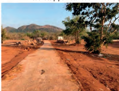
Access road construction
