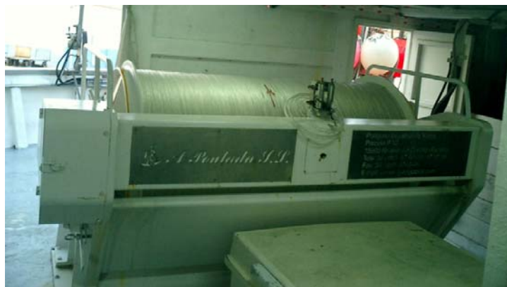
Figure 41. Hydraulic reel, where the mainline is stored.
